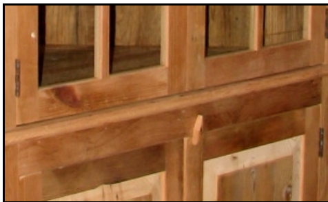
Cupboard lower cabinet doors are held closed by traditional hardware.
